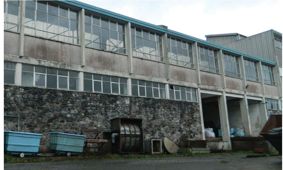
Figure 2.7 - Building E (View 2)
