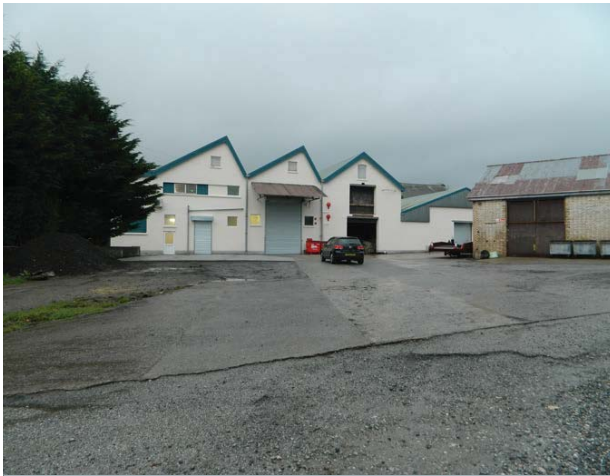
Figure 2.8 - Buildings Cx, Cy and F (View 3)
