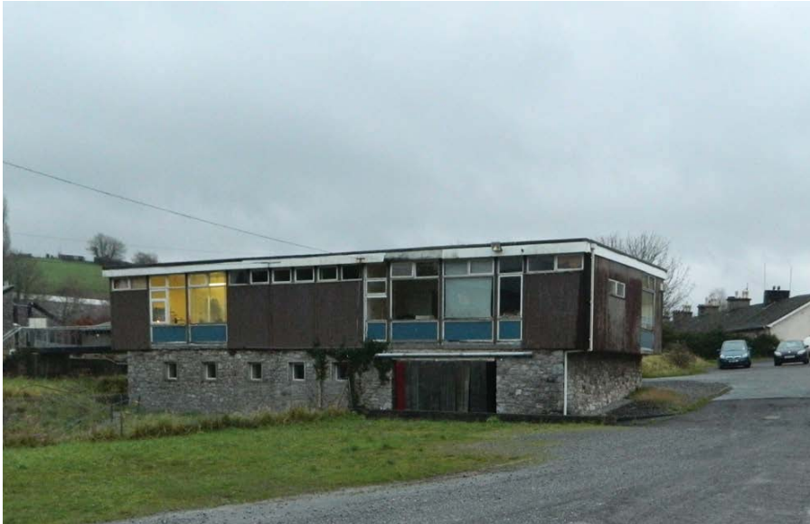
Figure 2.6 - Building A (View 1)
